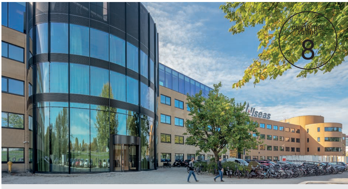
Renovation Allseas Office Delft
