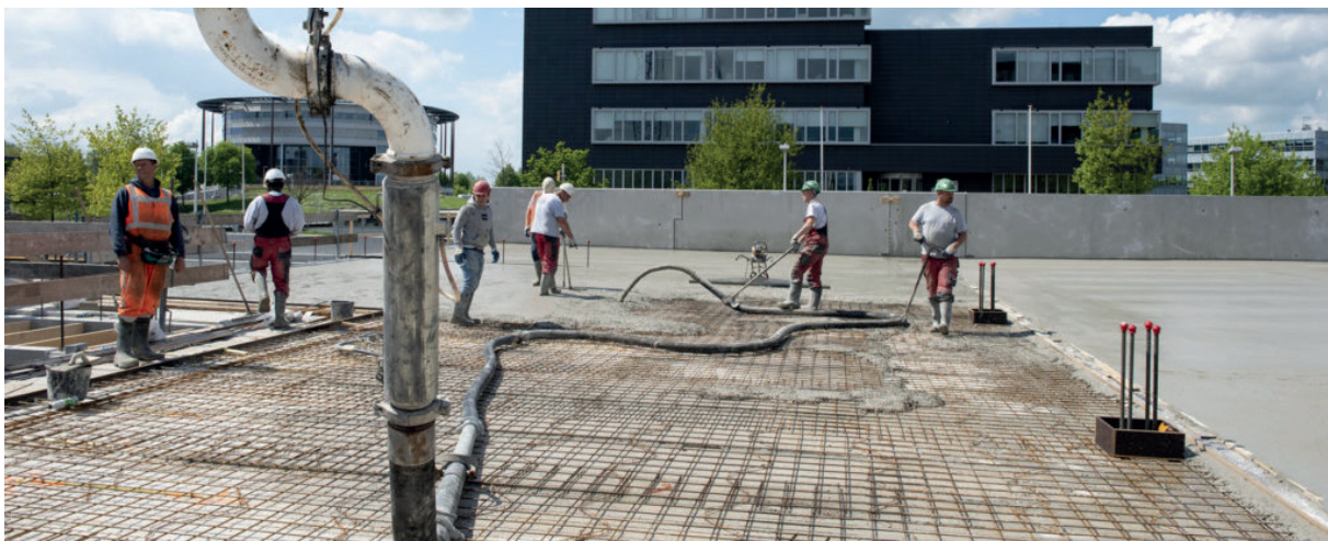
Circular concreting at NVM
