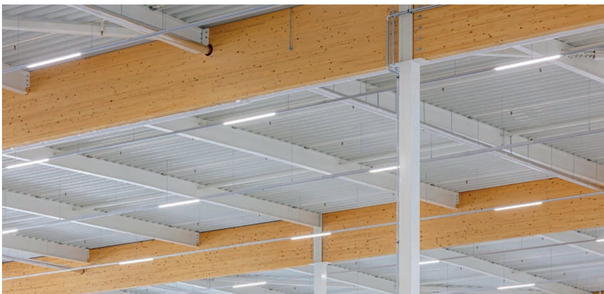
Roof structure of steel with wooden beams at Virgo Aalsmeer
