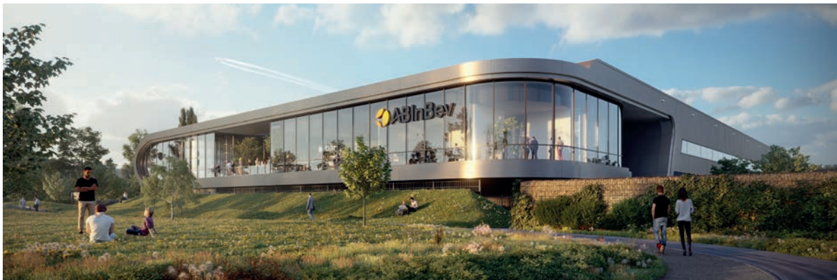
"State-of-the-art" urban distribution centre at Businesspark Amsterdam Osdorp for brewer AB InBev
