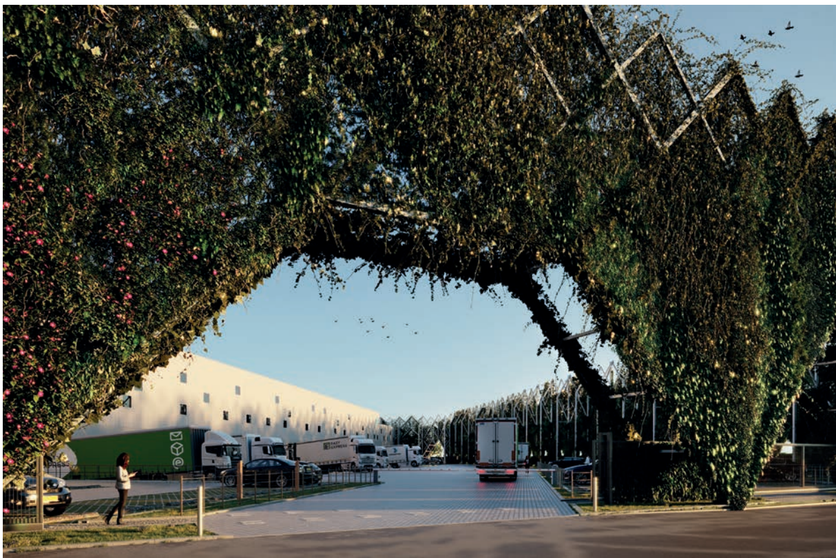
Ara Almelo's unique green facade (1 kilometre long, 15 metres high) was designed parametrically - Project Ara Almelo
